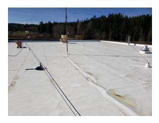
On the lower 1st story roof they added an anchor point at the ladder and another contractor cable that covers the smaller, lower roof level.
