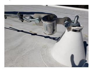
The antenna wires are also connected with anchor points so the contractor cable can be unclipped from the wire and attached at the antenna anchors for more roof coverage.
